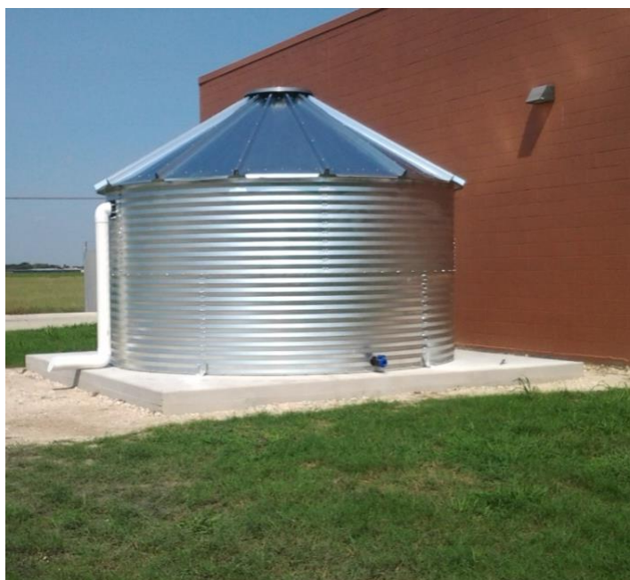
Figure 2. 10,000-gallon rainwater harvesting system at the Caldwell County Justice Center
