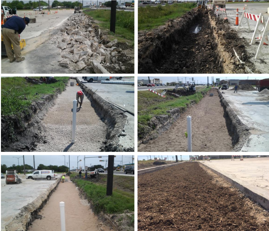
Figure 5. Construction of rain garden
