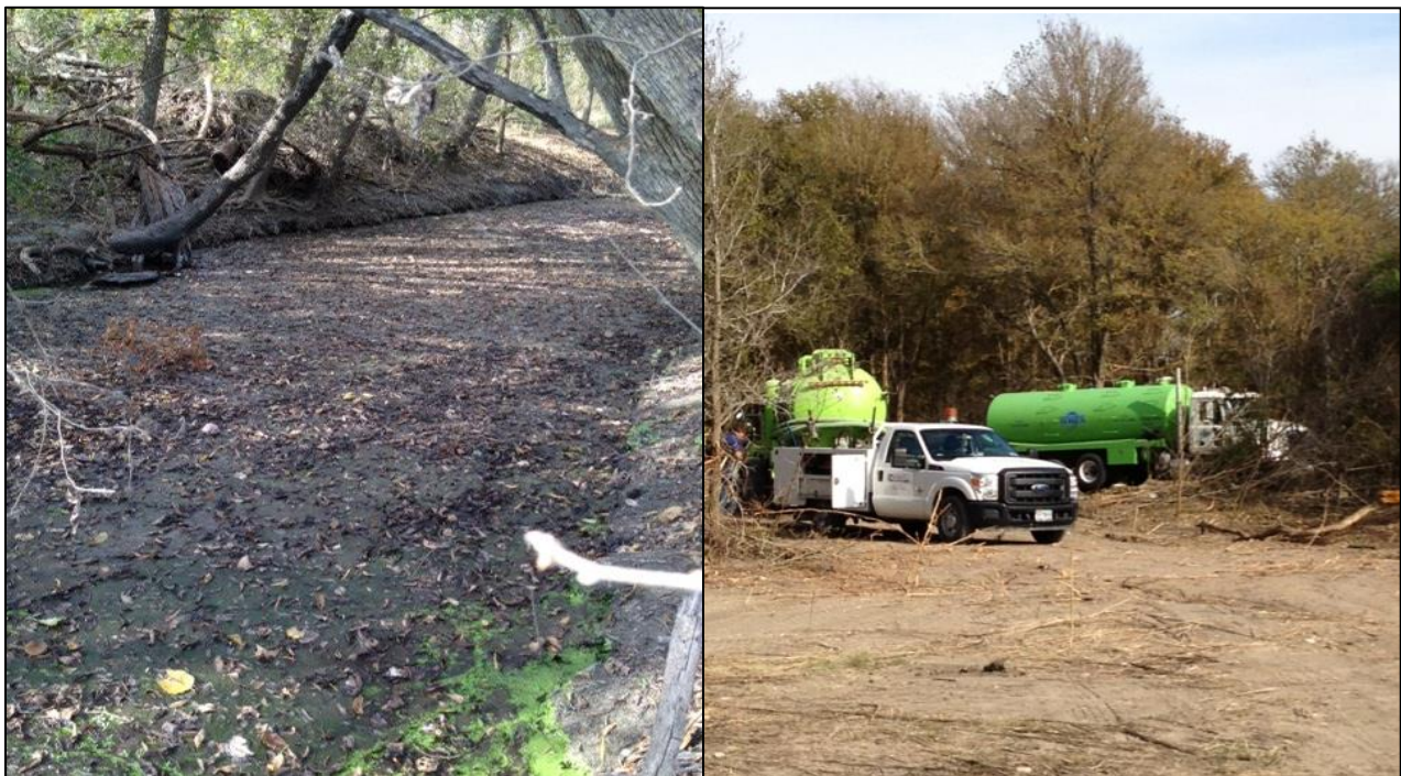
Figure 6. Sludge filling Plum Creek downstream from Kyle WWTF looking west from Heidenreich Road (left), Tankers pump sludge from Plum Creek near Kyle WWTF outfall (right), November 21, 2012. Note damage to riparian vegetation. Photos by Nick Dornak, WC
