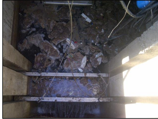
Figure 8. Sludge in wet well, Plum Creek Community Golf Course, Nov. 3, 2012.
