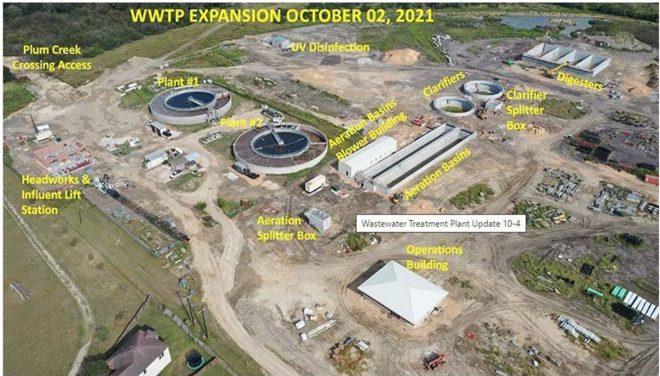
Figure 8. Progress of Kyle's WWTP expansion (2021).
