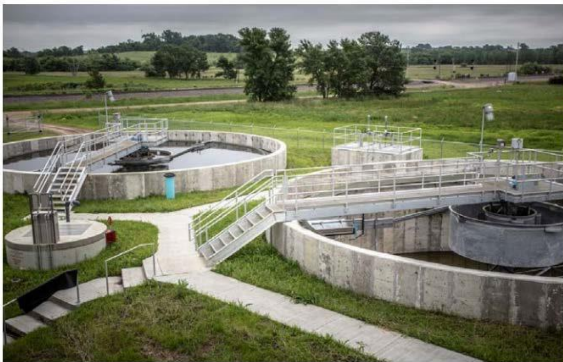
Figure 7. Example of a WWTP provided in the City of Buda Capital Improvements Plan 2018- 2022 , pg. 24.
